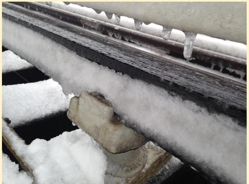
Ice buildup on a third rail along the NYCT Flushing Line
